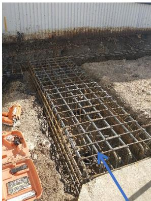
Beam attached to screw piles to disperse weight to foundations
